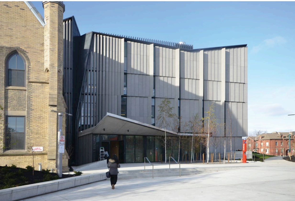
7. The fins cladding the exterior of the extension are repeated indoors as colourful stripes above the principal hall
