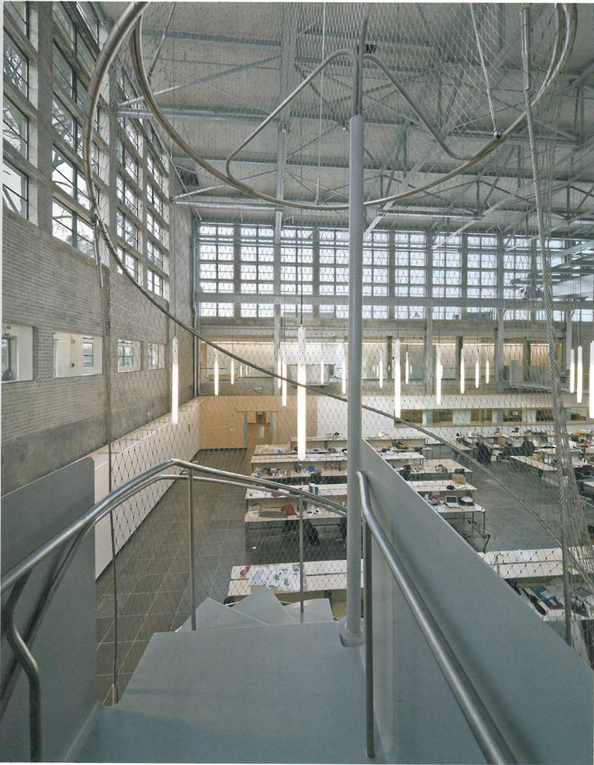
All images, unless otherwise noted: NADAA in collaboration with Lord, Aeck & Sargent, Hinman Research Building renovation, Georgia Institute of Technology, Atlanta, Georgia, 2011. Photographs: Jonathan Hillier
